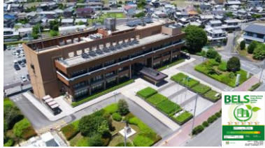
ZEB Ready acquired Kamigori-cho Town Hall Main Building
