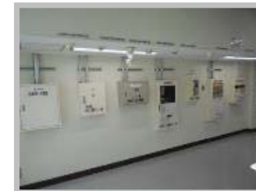
Haneda Safety Training Center Training using actual equipment (2)
