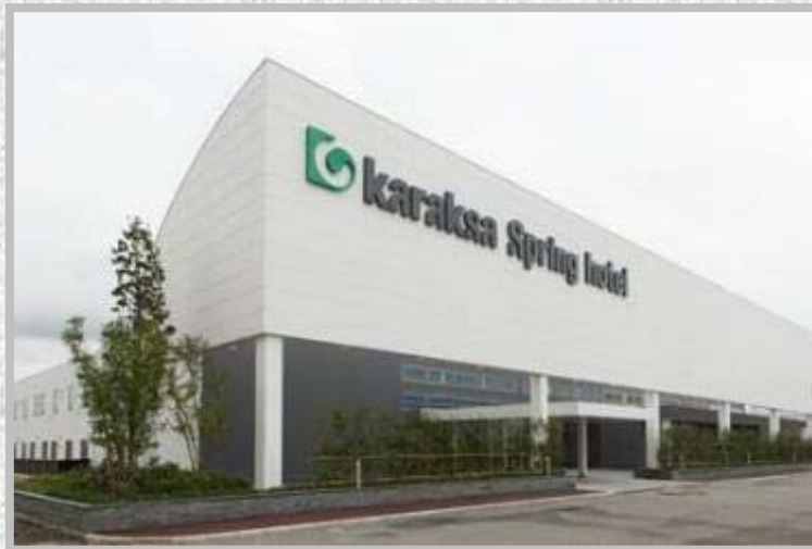
Conversion from electronics retail store to hotel
