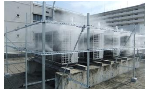
Spraying a dry mist over the rooftop air conditioning equipment
