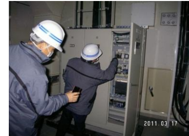
Repair work at a communication facility of the NTT Group
