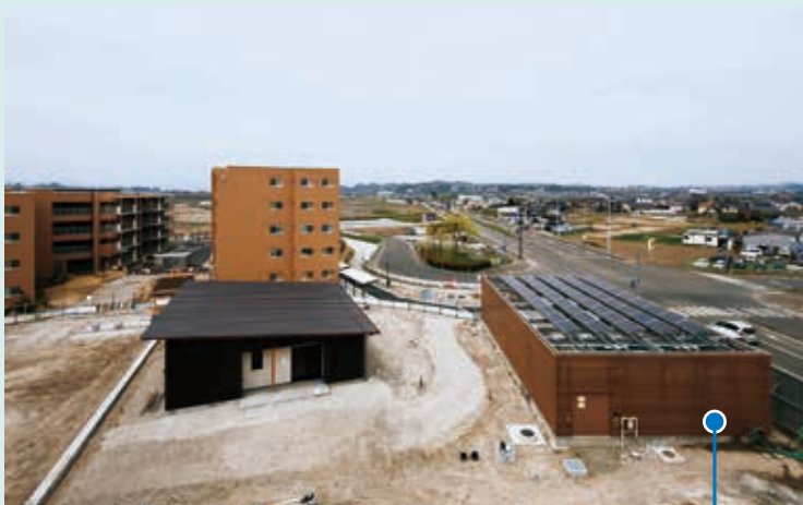
1. Sendai, Miyagi Prefecture 2. Energy center 3. Energy management system 6. March 2014
