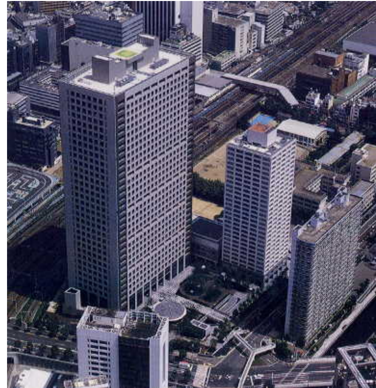
Tokyo Main Office (NTT Urban Development Grandparktower)
