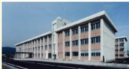
Koriyama General Prefectural Government Building
